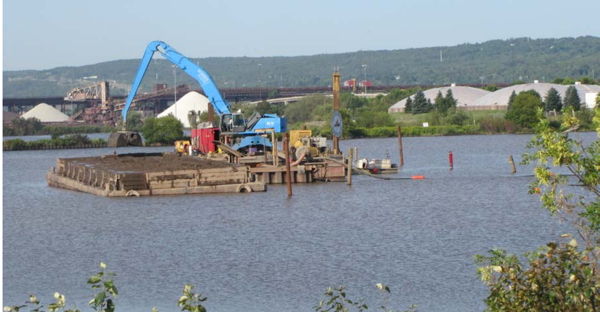
Contaminated sediment remediation in the St. Louis River, Duluth, Minnesota. Credit: Minnesota Pollution Control Agency.
