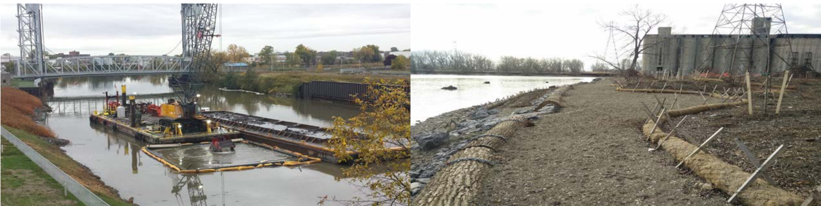
Contaminated sediment remediation in the Buffalo River (left), and shoreline habitat restoration along the Buffalo River (right). Credit: Buffalo Niagara Waterkeeper.
